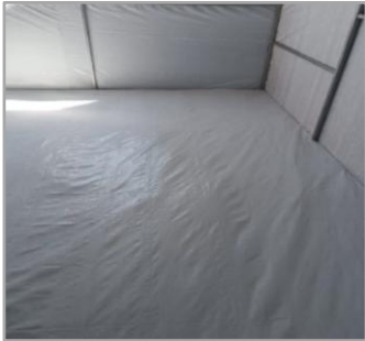
Figure6 Covering the floor with plastic tarpaulin
