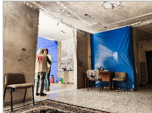
Figure7 Interior sealing off to walls inside the housing unit (source HEKS/EPER July 2025)
