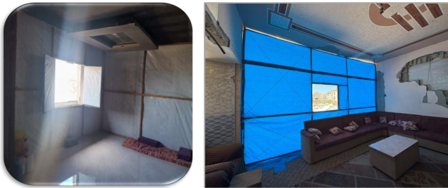
Figure2 Examples from Gaza of closing wall openings with tarpaulins
