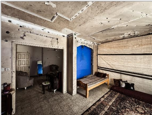
Figure7 Interior sealing off to walls inside the housing unit (source HEKS/EPER July 2025)
