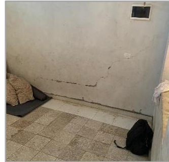
Figure5 Replace the damaged area with reclaimed tiles
